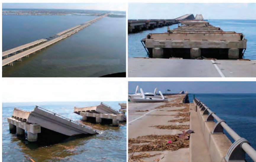
FIGURE G-25 Lake Pontchartrain Bridge damage from Hurricane Katrina.
