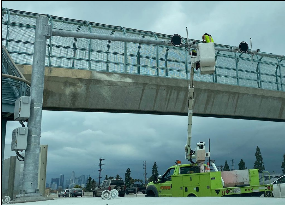
Installation of cameras and illuminators on the ODS overhead gantry at the I-110 North location
