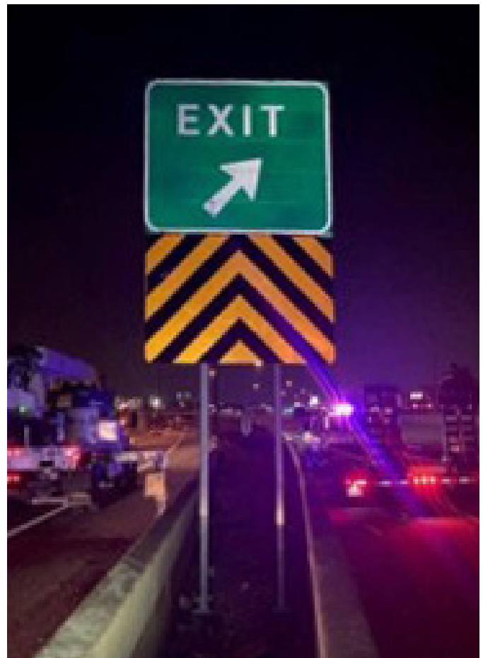
FIGURE 4. Reflective chevron sign improves Exit signage visibility, especially at night.
