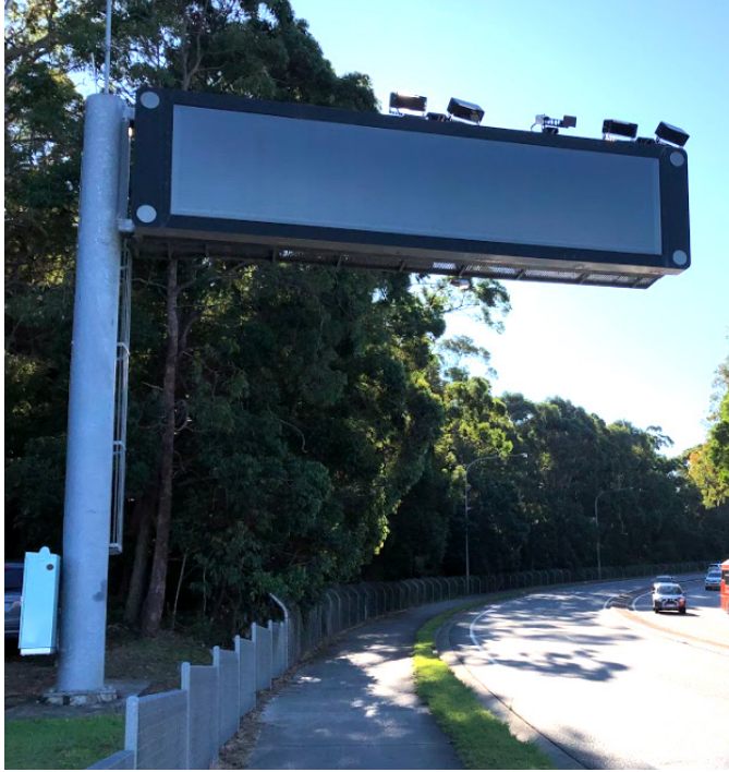
FIGURE 1. High-definition infrared camera systems can be mounted on an existing gantry to establish network-wide behavioral baselines.
