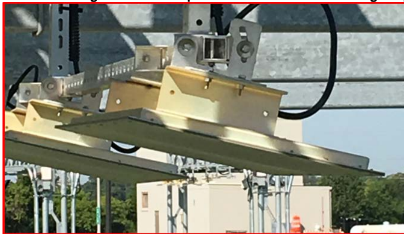
Figure D-1: Example of antenna installed on a gantry
