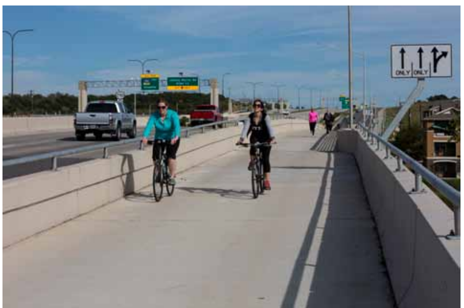
290 Toll (Manor Expressway – top) as well as the adjacent shared use (hike and bike path – above)
