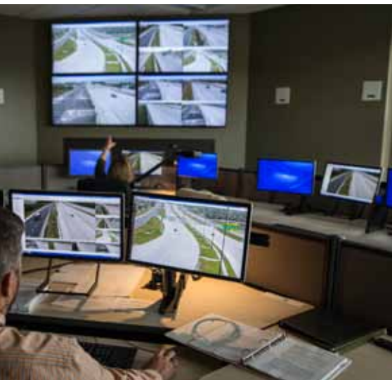
This operations center will be the control center for the MoPac project
