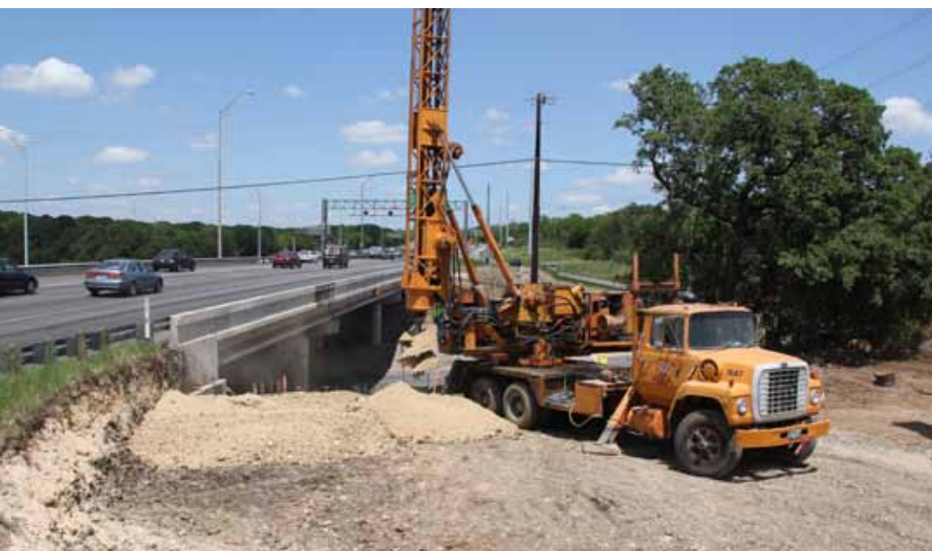
Construction of the MoPac Express Lanes
