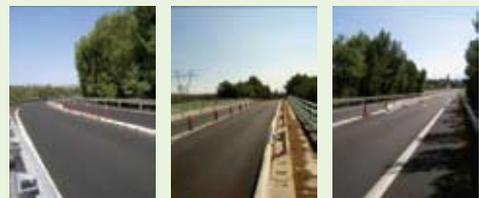
Figures 2–4: The French motorway network employs a combination of mini-GBA (glissières béton armé), or reinforced concrete, systems and mini-BOA (barrières ouvrages d’art), or protective barrier, systems to help prevent ghost driver incidents.
