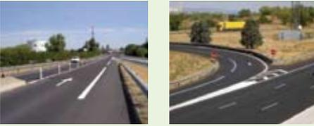
Figures 5–6: Directional arrows painted on the road indicate the correct (left) and incorrect (right, with no-entry signs) paths.
