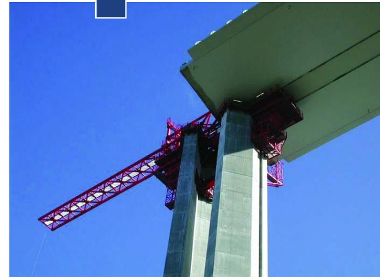
with each 171-meter section taking around four weeks to assemble. With very strong winds in this part of France, section assembly over the void might have proved hazardous. The gradual overhang method, however, meant that the only weather requirement would be low wind speed (below 85 km/h) during the two days each section was pushed out (i.e., every four weeks). The schedule would therefore suffer minimum interference from weather conditions.
