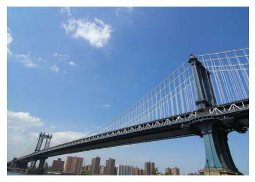
anchorages, towers, main cables, and suspender ropes, which are not found on a truss span.
